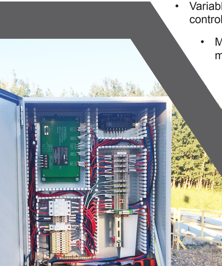
CROSSFIRE Controller Installed in Electrical Panel
